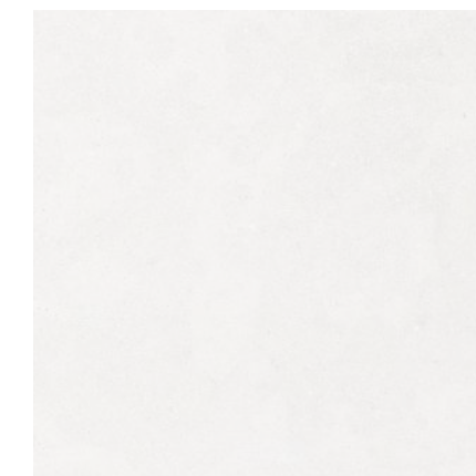
Internal walls in warm white clay plaster.
