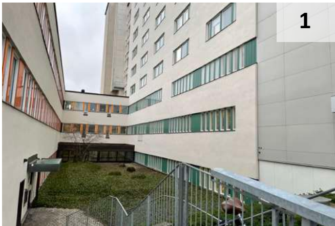
Courtyard between buildings in the north
