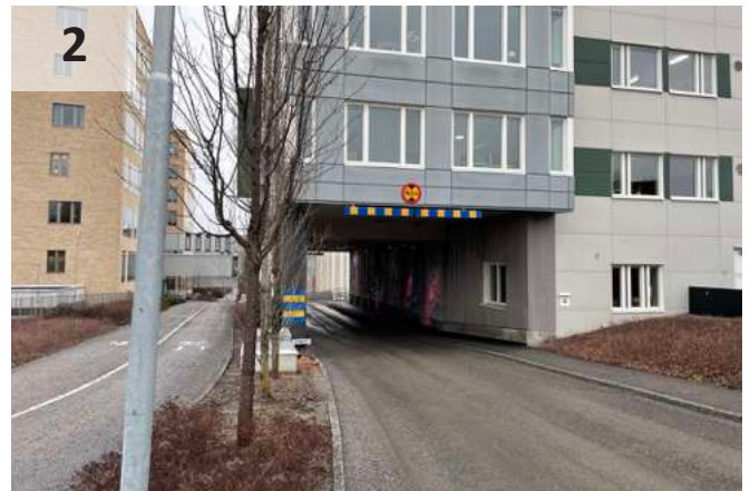
Road under house 85- NIMA & NIVA in ground level
