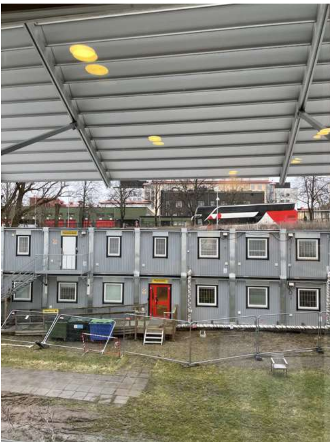
View from care room with exterior sun shading
