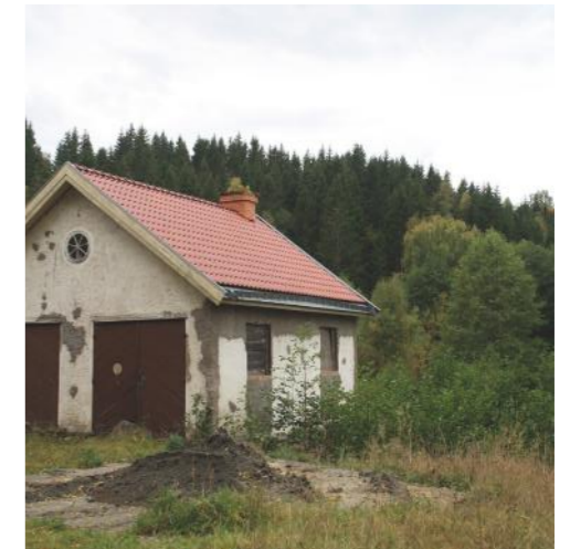
Fig. 33. Former garage, Strömsfors, 2022
