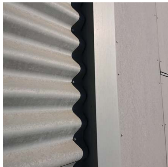
Corrugated metal sheet. Own photograph from Innovatum
