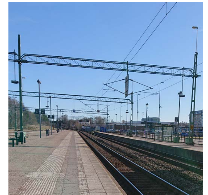
Trusses by train tracks. (Own photograph)
