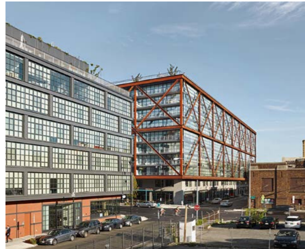
Figure 13. Atlantic Plumbing (Morris Adjmi Architects, Karchmer A., n.d.)
