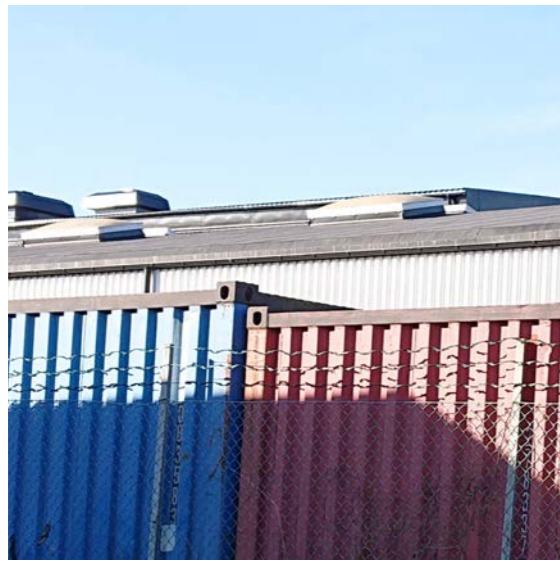
Corrugated metal plates. Own photograph from Ringön.
