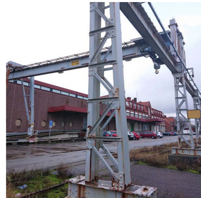
Traverse next to the carriage workshop. (Own photograph)
