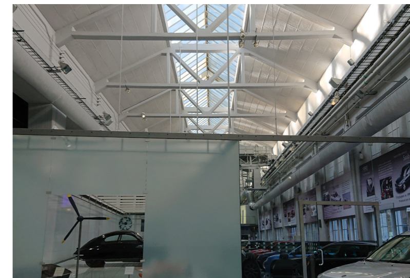
Dividing wall of frosted glass compromising the effect of the axis of the building. (Own photograph)
