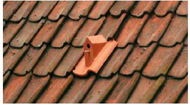
Figure 16. Bird roof box.
