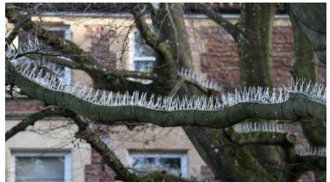
Figure 3. Installed anti-bird spikes.
