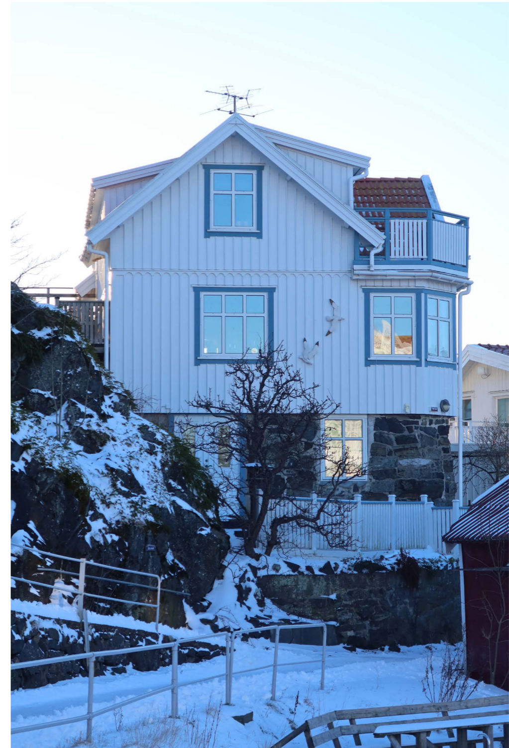
Additions to a villa on Åstol. The clear shape of the original villa makes it still readable despite multiple additions.
