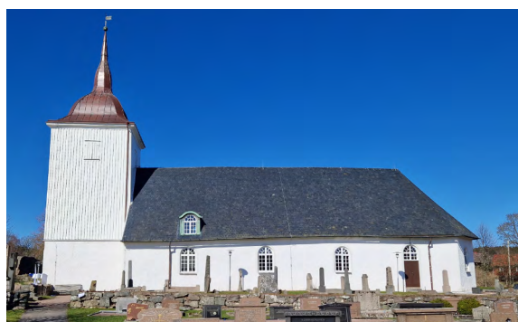
Säve Church. The central part is thought to date to the 1200s, while the rear and tower were added in the 1700s.
