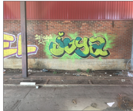
Fig. 62. The uncontrolled: traces of 'illegal' activities next to Kallförrådet, Lundbystrand.
