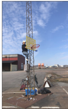
Fig. 116. On site preparation for mounting the hoop board.
