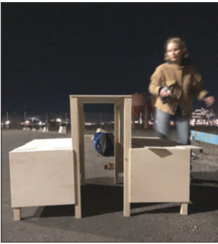
Fig. 79. Building on site.
