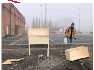
On-site alterations (repairing, painting) of design experiment Traversings.
