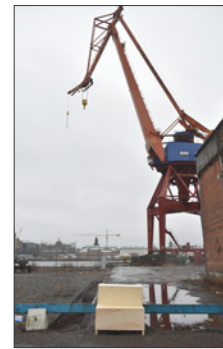
Fig. 90. New sequence (D). Staircase structure traversing low concrete barrier.
