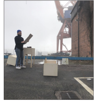
Fig. 94. Repairing the stairs.
