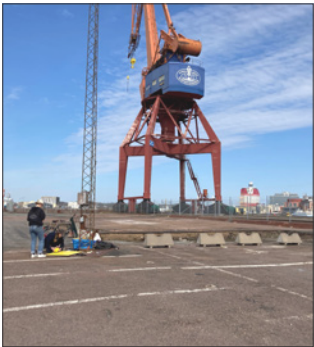
Fig. 115. On site preparation for mounting the hoop board.
