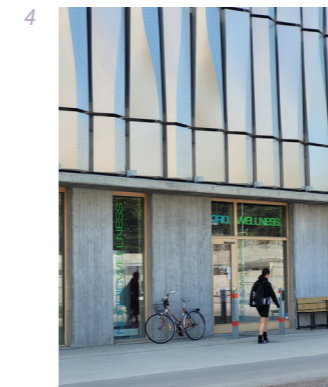
Along the main street there is a big gym in the bottom floor
