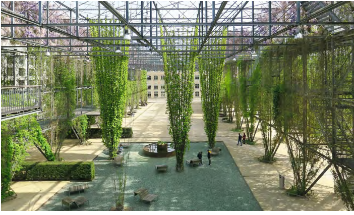
Fig 21&22. Interior and exterior of building structures MFO Park, Zürich
