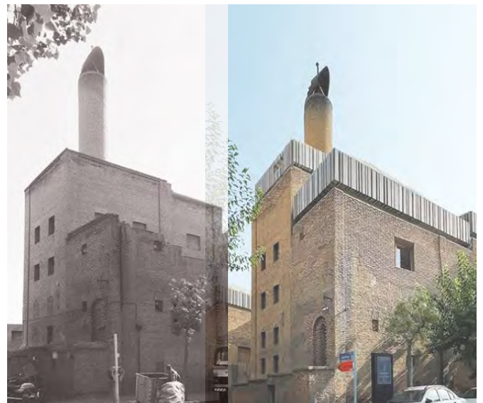
Fig03& 04. Argo factory (Before and after), Tehran, IR
