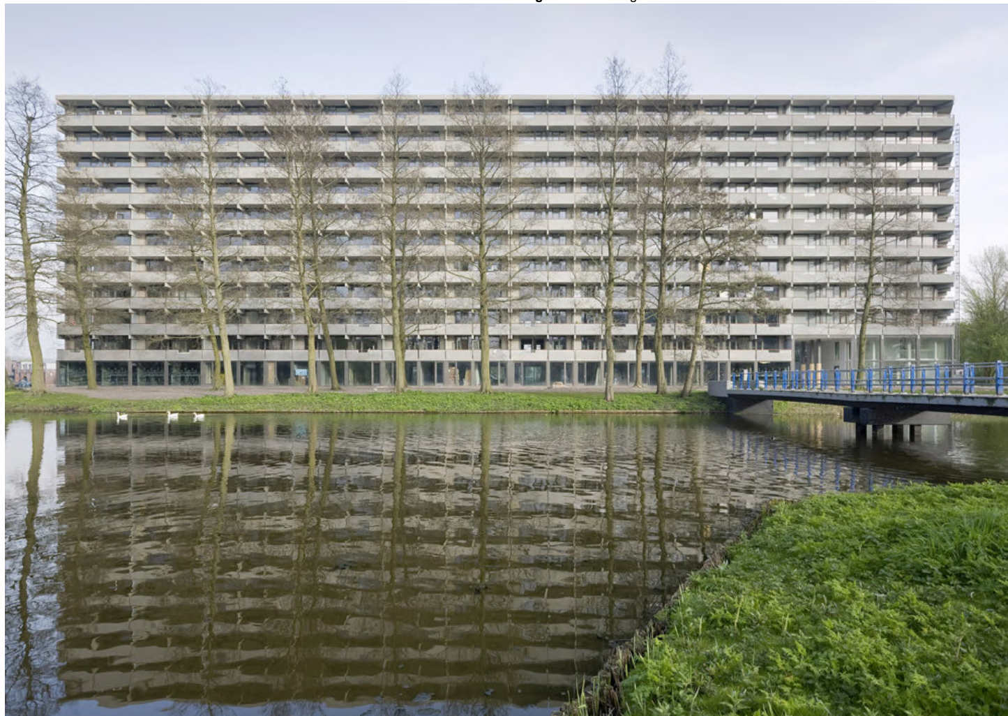
Figure 24: Building entrance and facade
