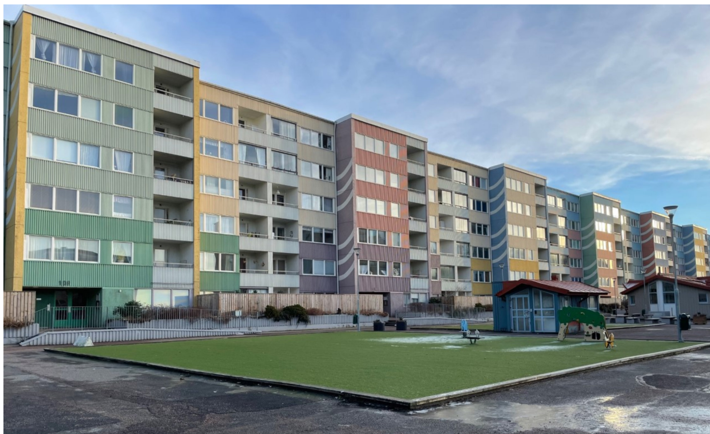
View over yard and building in the area
