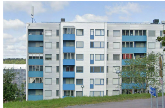
The facade after the renovation
