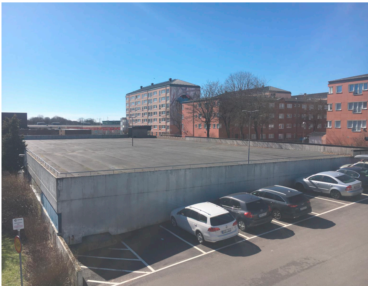
Picture of the parking lot from the north bridge
