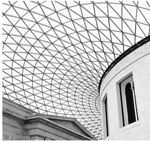
Figure 4. British Museum Great Court is one of the most prominent examples of a gridshell in steel by Buro Happold with Fosters + partners.
