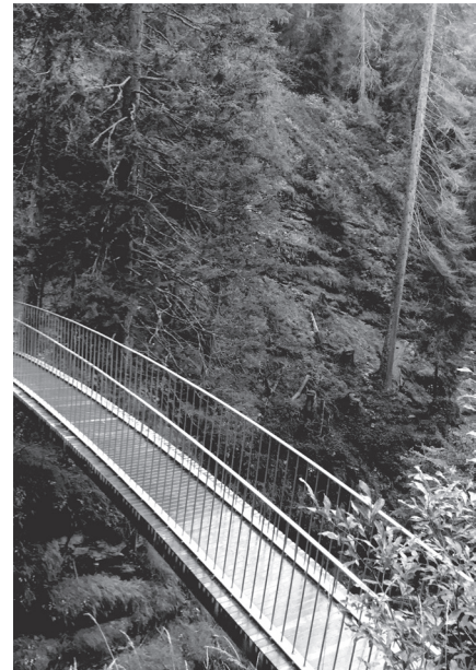
Figure 81 Wasserfallbrücke by Jürg Conzett, one of seven bridges along the Trutgdil Flem, a hike along the Flem River in Switzerland.
