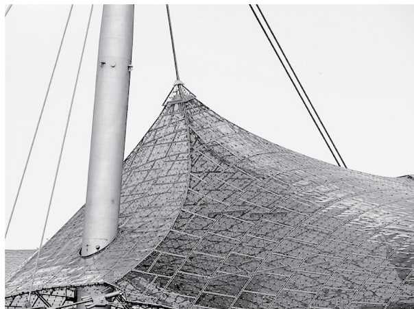
Figure 9. Tensile structure for Munich Olympic Stadium (1972).
