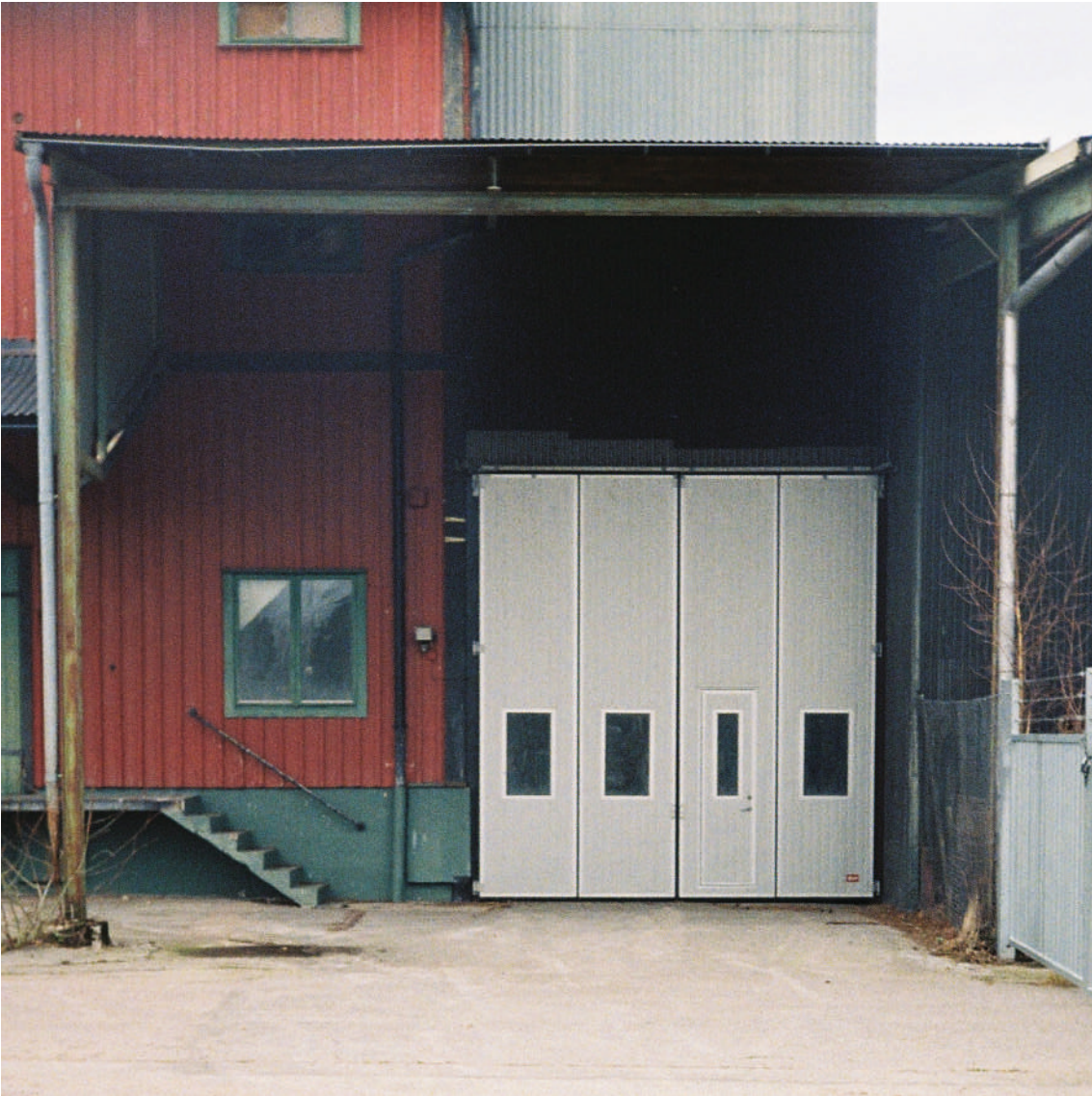
The entrance to the silo
