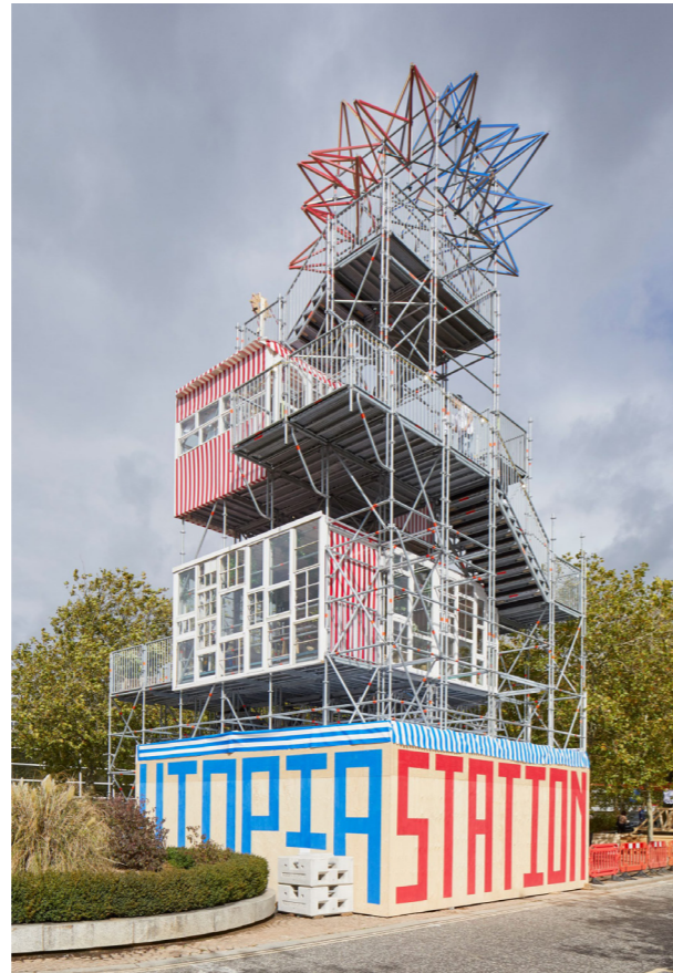
“The Built, The Unbuilt and The Unbuildable” Pavillion by raumlaborberlin in England. Image: raumlaborberlin, 2019
