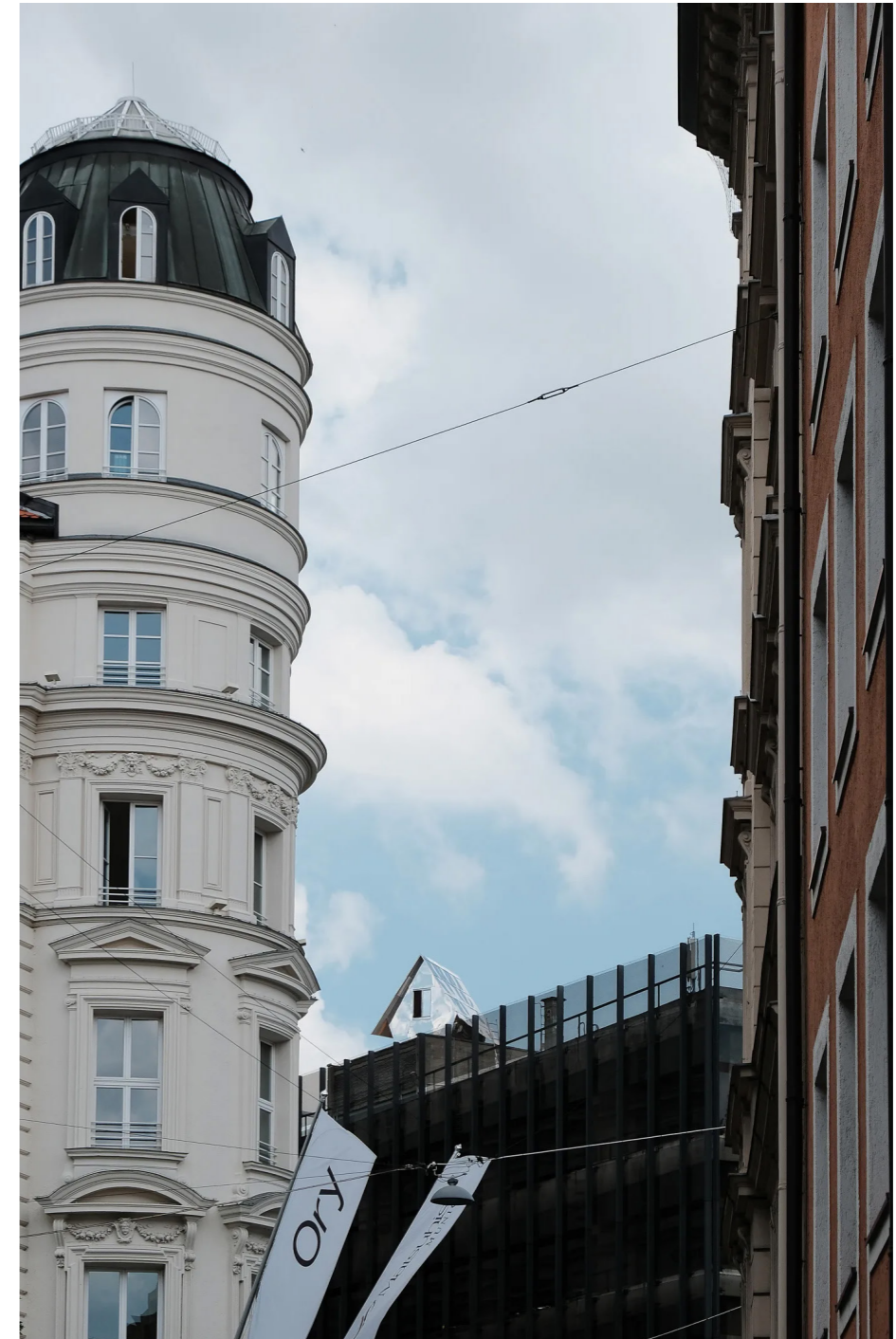
The “Penthaus à la Parasit” on top of a parking garage in central Munich.
