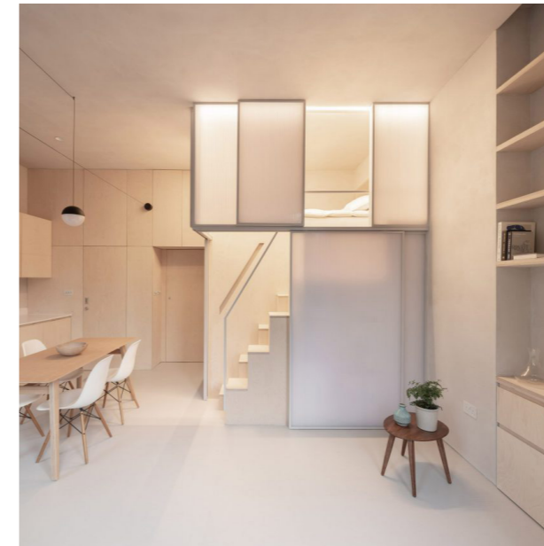
Figure 29. View of the function box attached to a wall with transparent panels in the sleeping area on the loft.
