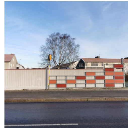
Walls to protect the neighborhood from noise
