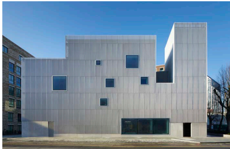
Figure 1.3: Energy Hub [Jack Hobhouse]
