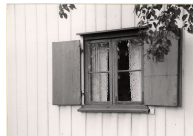
Figure 2.14 The windows shape (© GhmD_16984, 1940)
