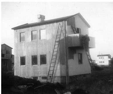
Figure 2.12 Facade of building type A (Bräcke småstugeförening, 1934)
