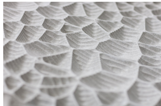
Figure 14, CNC-milled gypsum panel for the Elbphilharmonie Hamburg by architects Herzog and DeMeuron. Image from Hasenkopf Industrie Manufaktur
