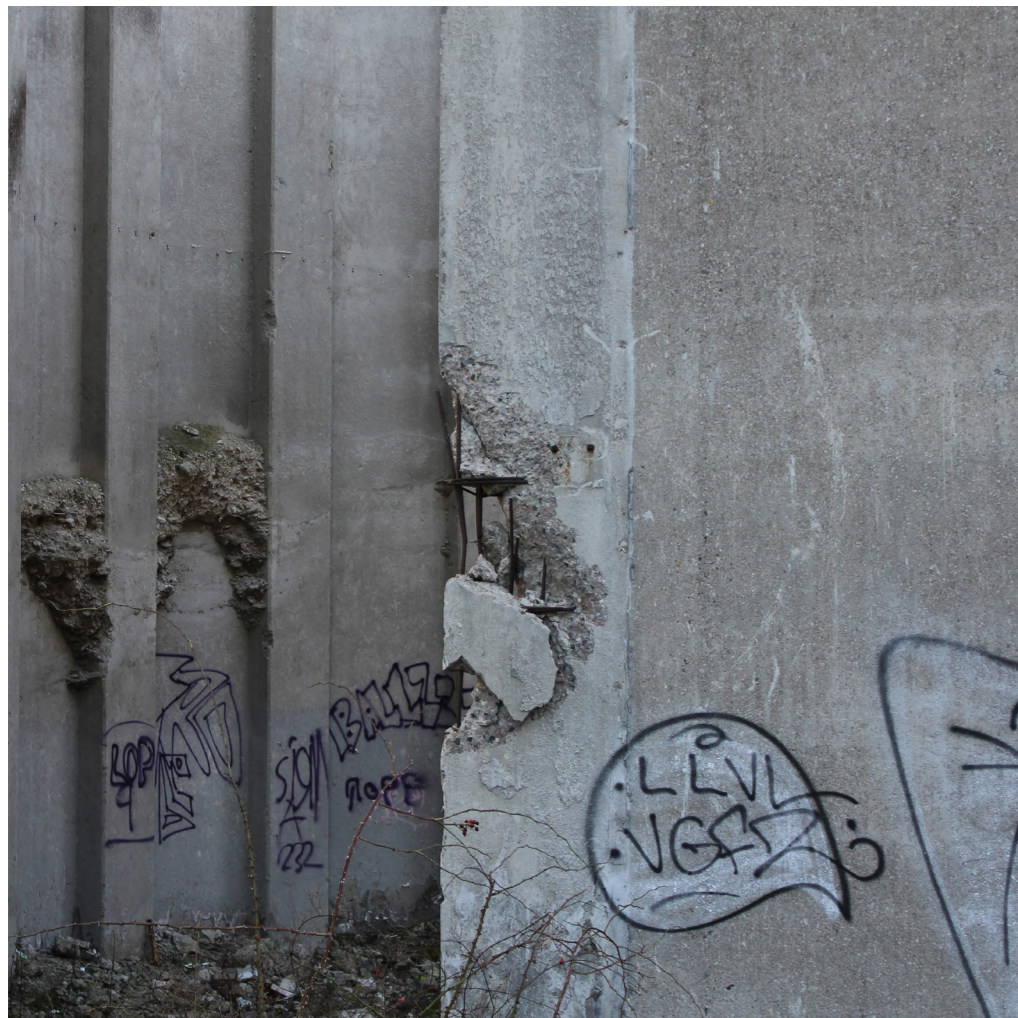
TOP LEFT MARKS AND TRACES OF FORMER CONNECTION BUILDINGS AUTHOR'S PHOTOGRAPH (2023)
