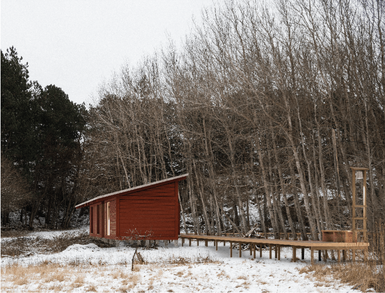
Fig. 28 NW facade and footpath
