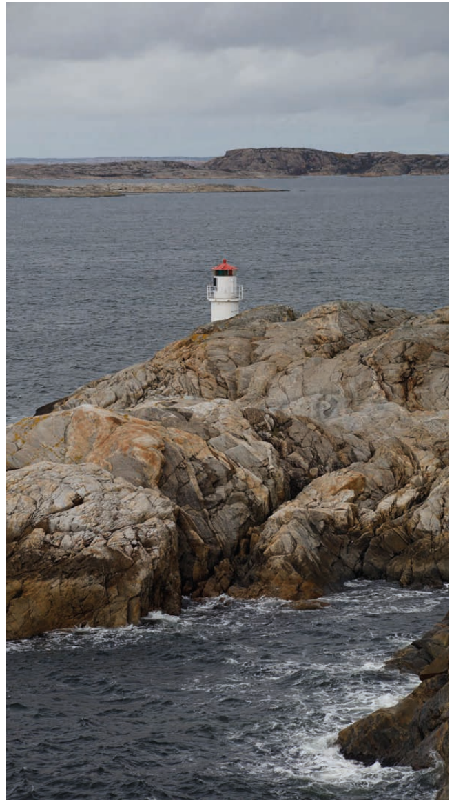
Fig. 01 New lighthouse at Torskepallen, Islandsberg
