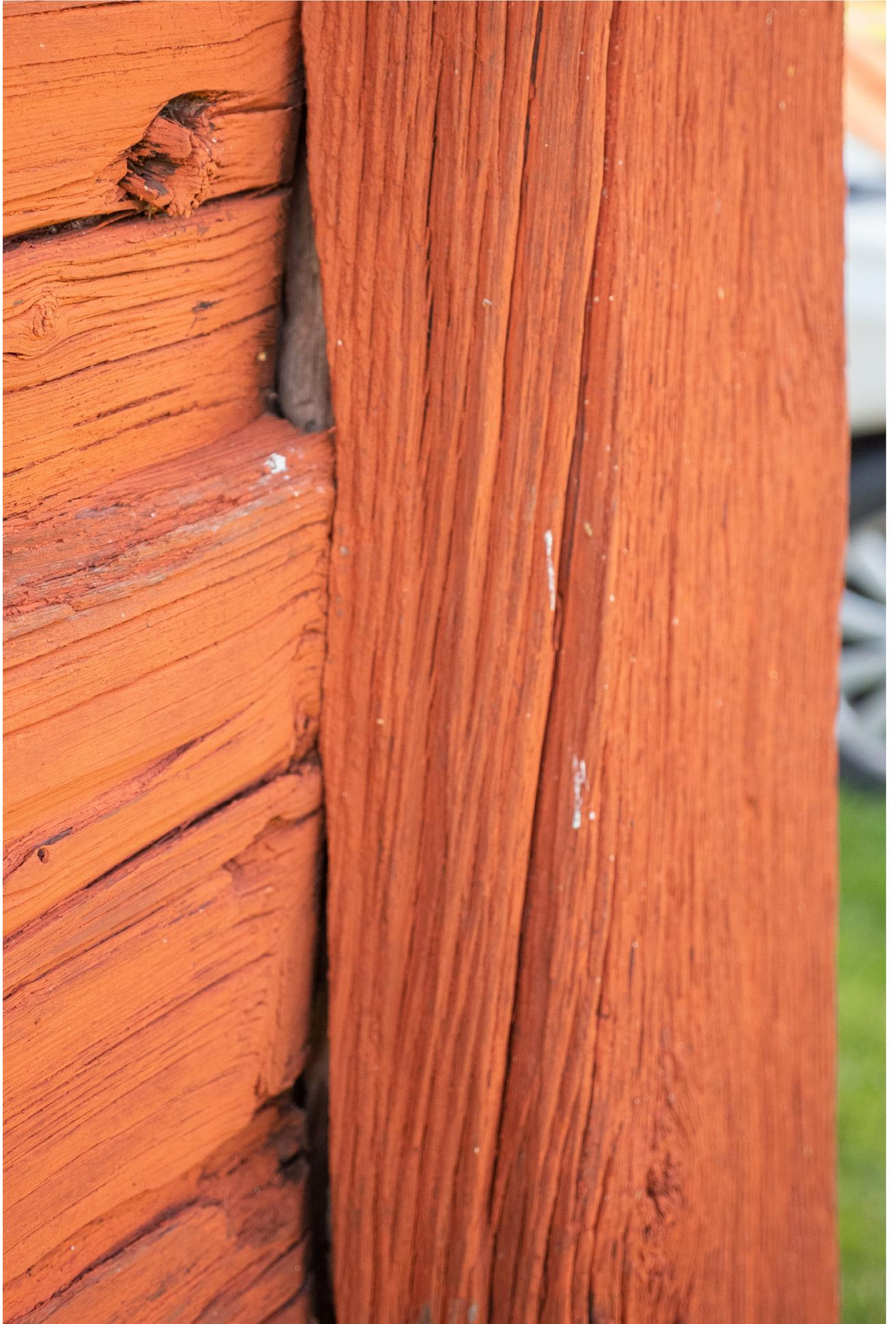
**Post and planks is a skeletal construction of timber and is therefore a flexible construction method that is honest and understandable as a structure. The skeletal construction enables working with precision in details as well as being flexible in both outlining the floorpan but also changing the infill from a full timber construction into a half timber construction that still shows the honest skeletal timber structure.**
