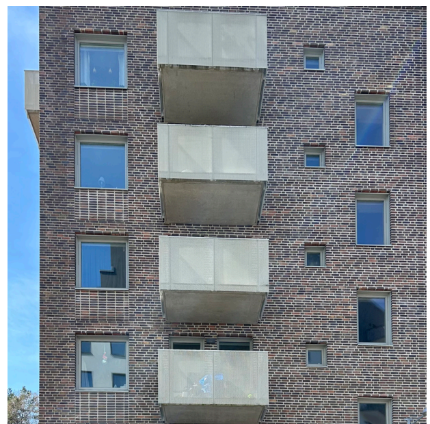
Fig. 27. Image facade, Flatås park.
