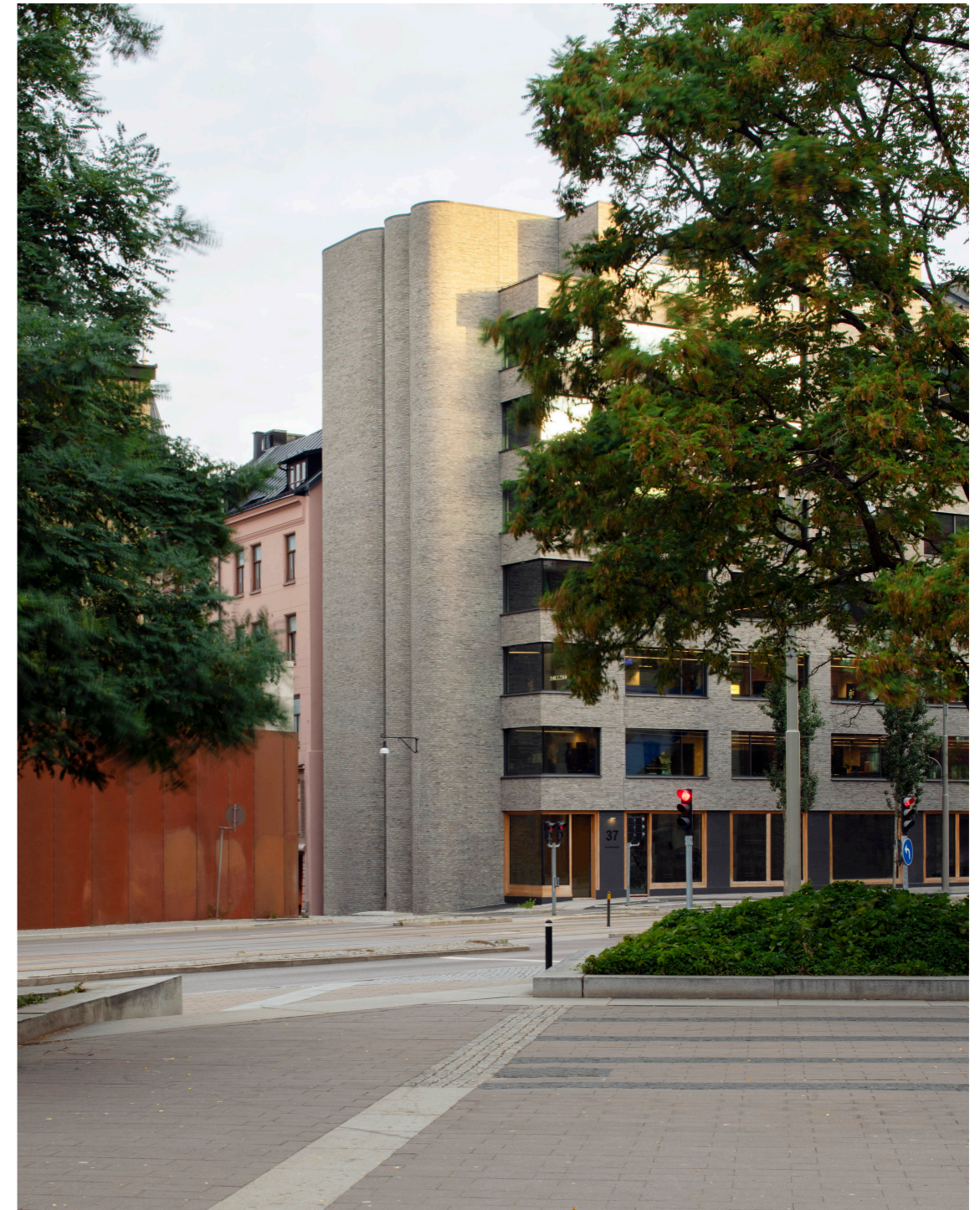
Figure 18. Facade with newly manufactured bricks (Olsson Lyckefors, n.d)
