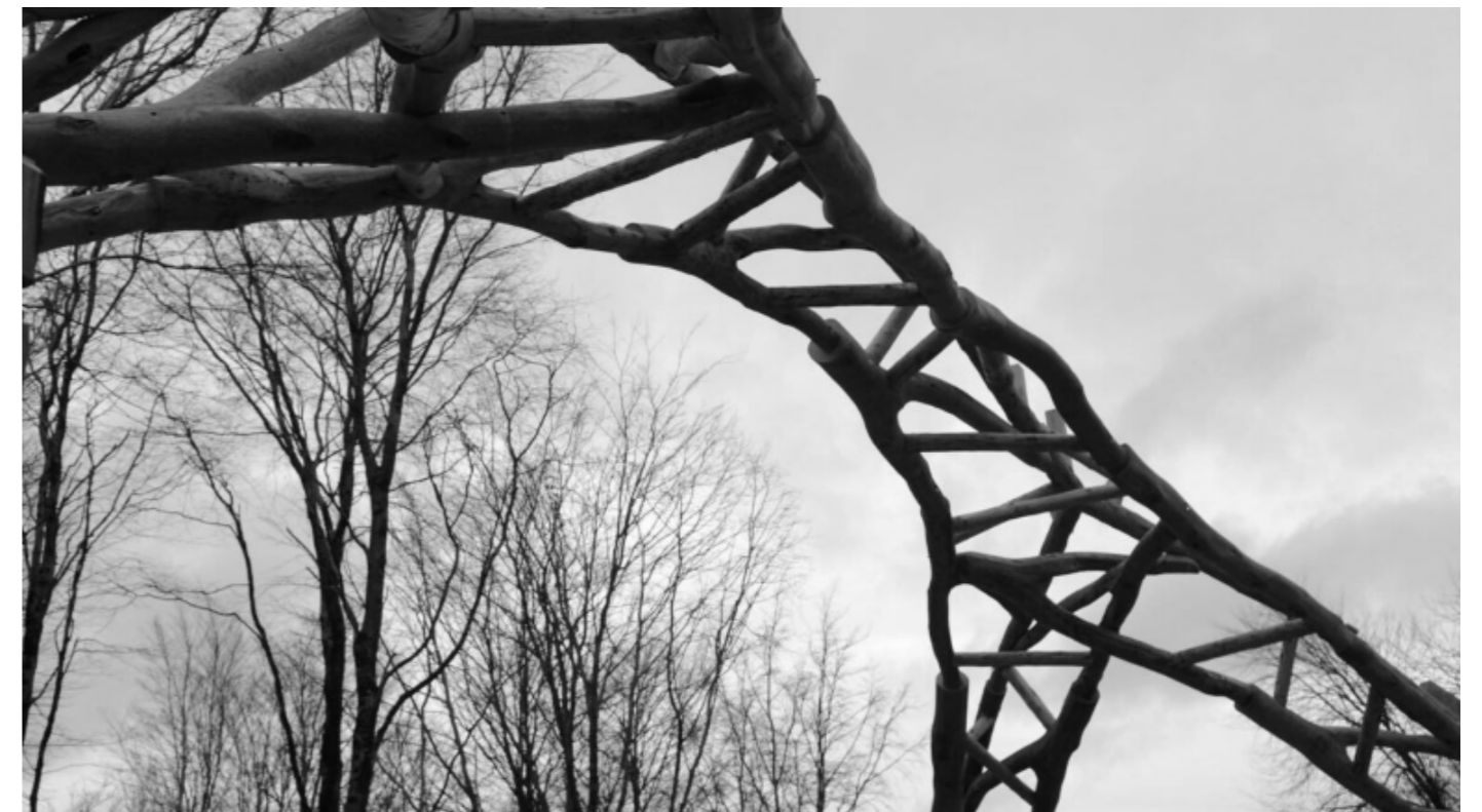
Fig. 7. The Tree Fork Truss.
