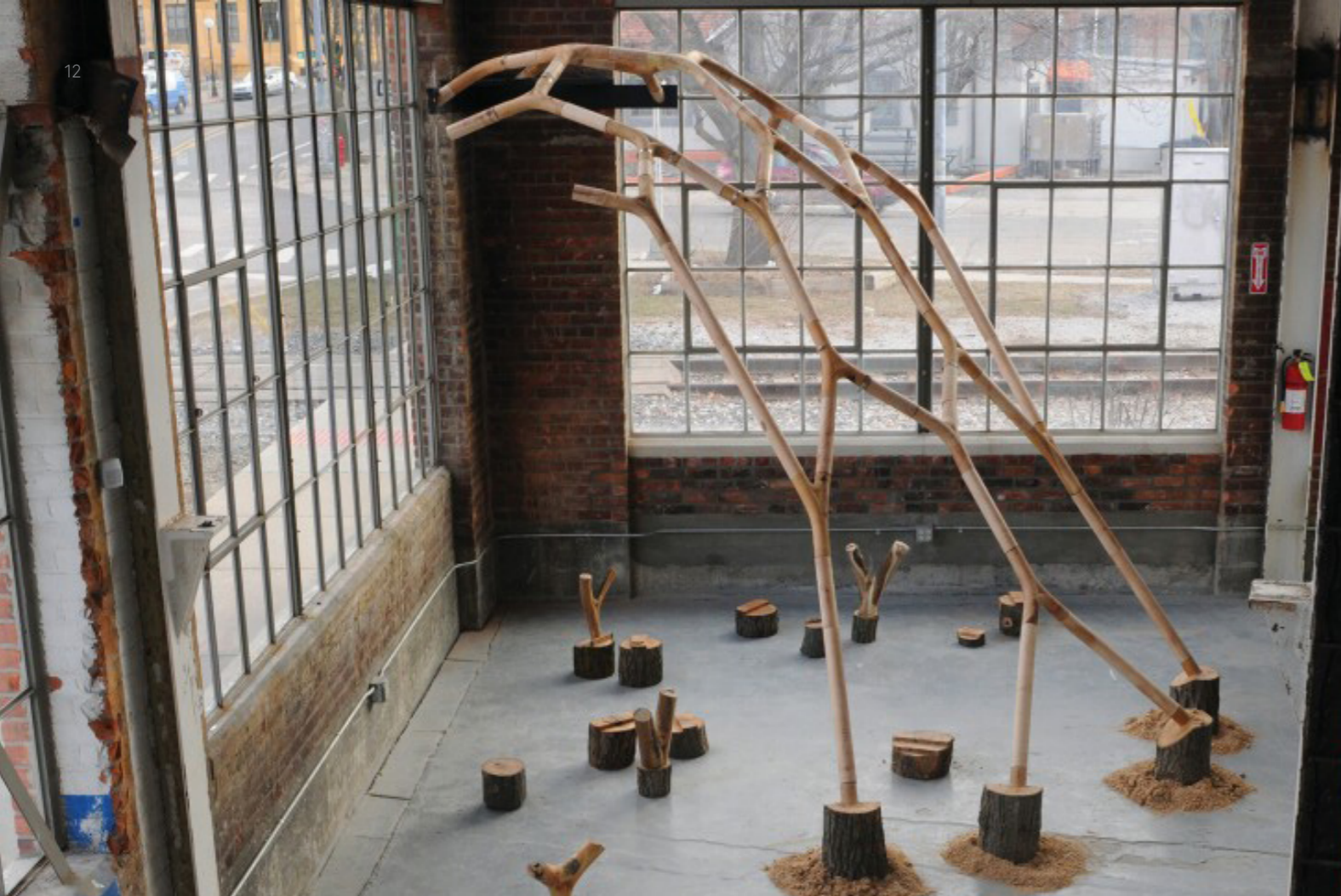
Fig. 8. Limb . Full-scale installation of one leg of a three-legged reticulated shell structure.
