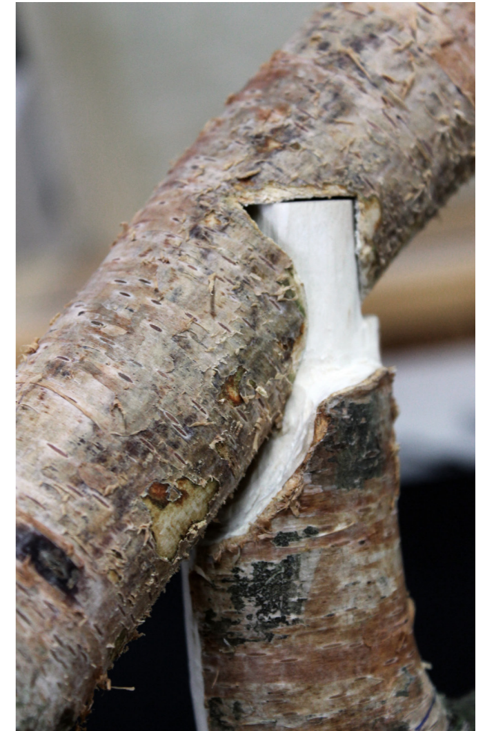
Fig. 66. Close-up of milled connection.
