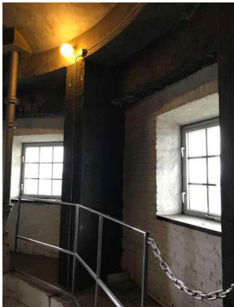
The level under the water tank
