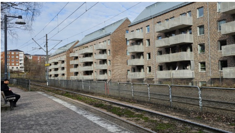
Figure 22b. Residential blocs near the tram tracks. Large windows allow strangers to view the interior of the apartments from the tram and the tram stop. The ground level is also placed lower than the tram tracks. The balconies are facing west, which is pleasant, but the noise and trams could disturb the experience..
