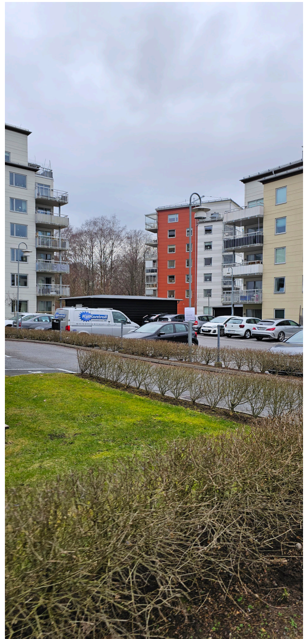
Figure 19b. One of the many parking lots between the tower structures, clearly indicating the dominance of cars.
