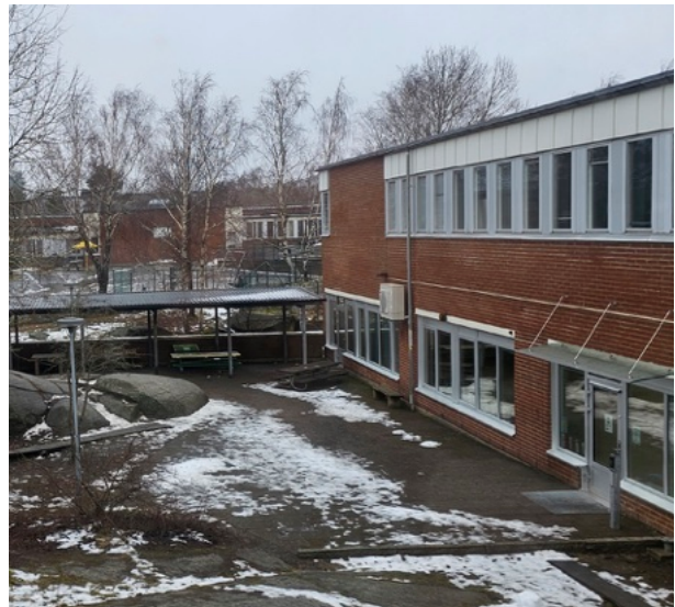
Figure 34a: Red brick facade, white lintels and continuous ribbon windows. The windows on the ground floor were changed in 2021 and the ones on the first floor were changed in the 1980's.
