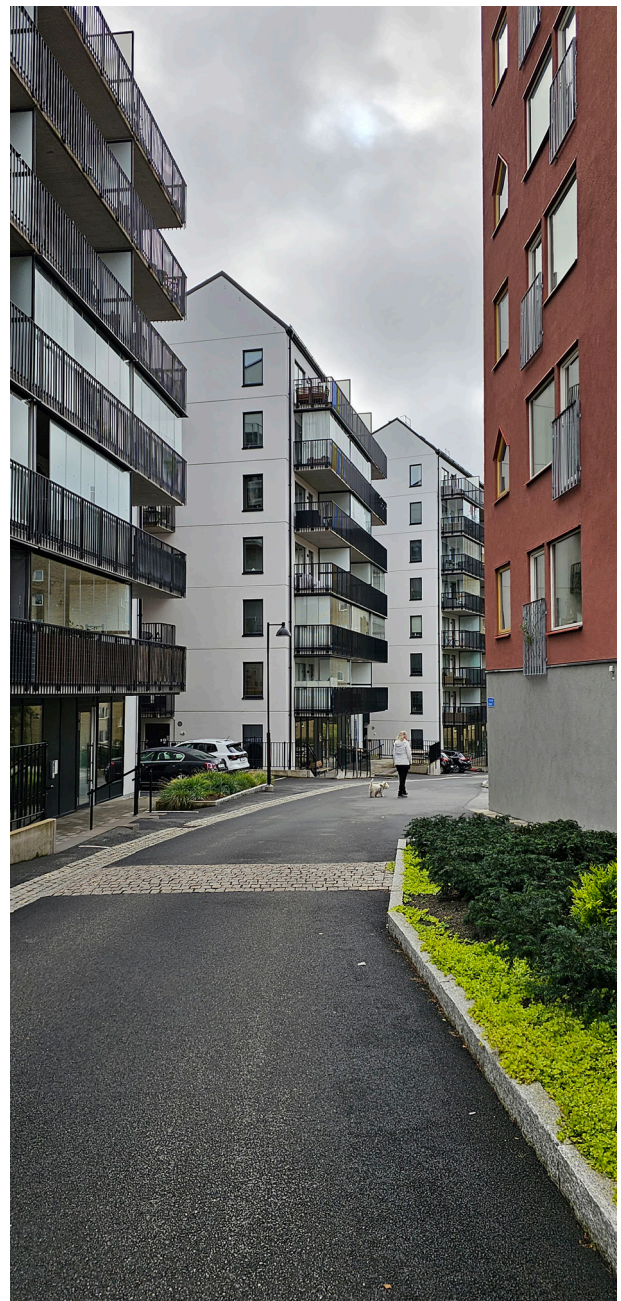
Figure 20a. Narrow one-way street separating the tower structures from the apartment blocks. Privacy issues as the neighbors will have free view into each other's apartments.
