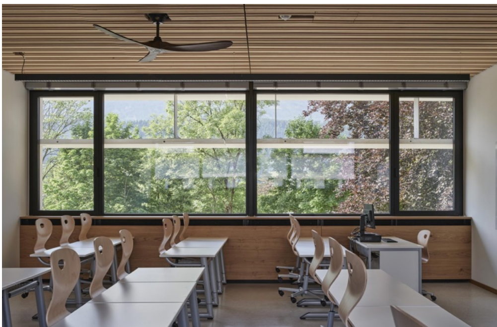
Figure 29b: Picture showing the classroom. The wooden box below the windows is where the trickle-vent is located. The fan on the ceiling further enhances the air quality during the warm summer days. Picture: Günter Richard Wett
