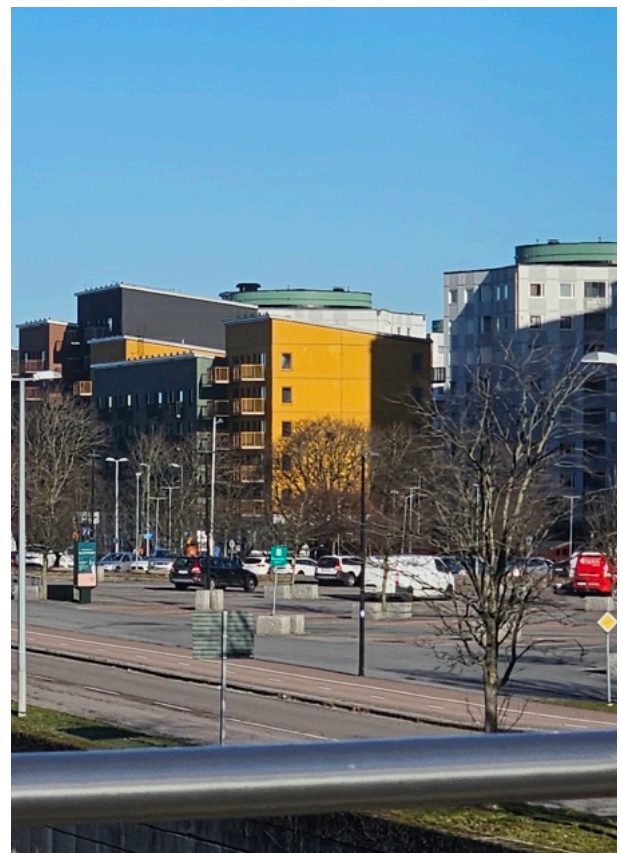
Figure 14. Picture of new urban densification project in Frölunda, with high exploitation numbers, under construction. The buildings are being placed close to existing structures. Is this the type of densification we will see on the grounds of Tynneredsskolan?
