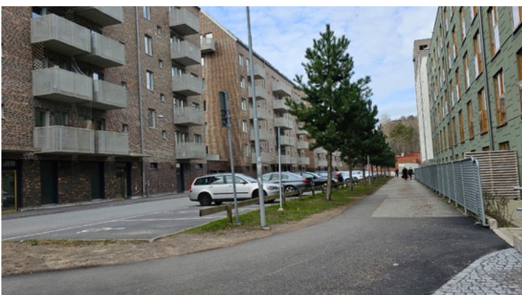
Figure 22c. Ground floor on the buildings to the right seems like commercial spaces at a first glance, but is actually parking spaces within the buildings. The building to the left have privacy issues, like other new buildings in the area. Many of the blinds were down at the time of the visit.
