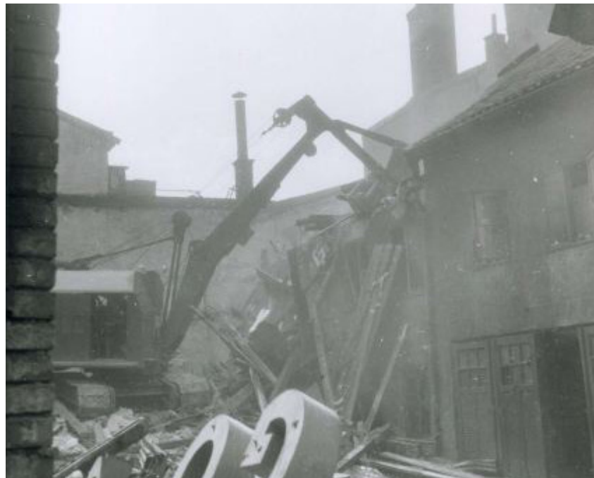
Demolition of Nordstaden
