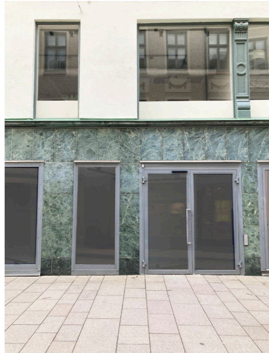
Fig. 53 Picture showing facade of building.
