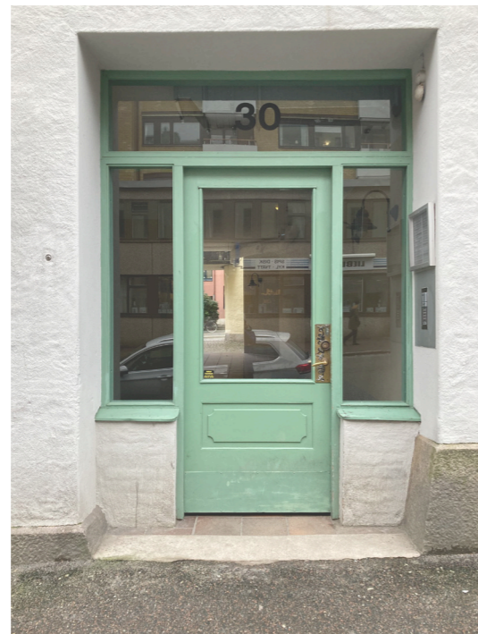
Fig. 32 To the left: The door towards the street leading into the portique.
