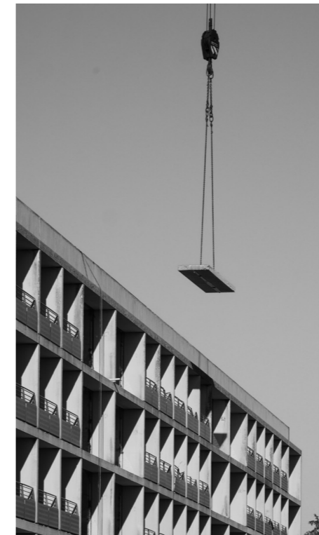
Fig. 5 Dismantling of HC element. Image source: GXN
