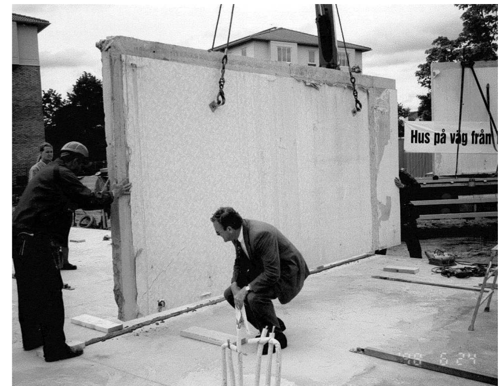
Fig. 3 Assembly of new building in Link ping. Image source: (Eklund, Dahlgren, Dagersten, & Sundbaum, 2003)
