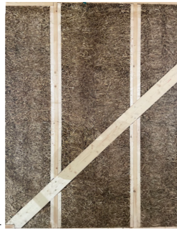
Image 1. The barn - "factory" Image 2. Pressed straw bale Image 3. Section of prefab panels
