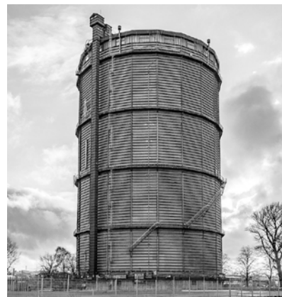
Gasklockan at the Gullbergsvass gasworks, Gothenburg.
