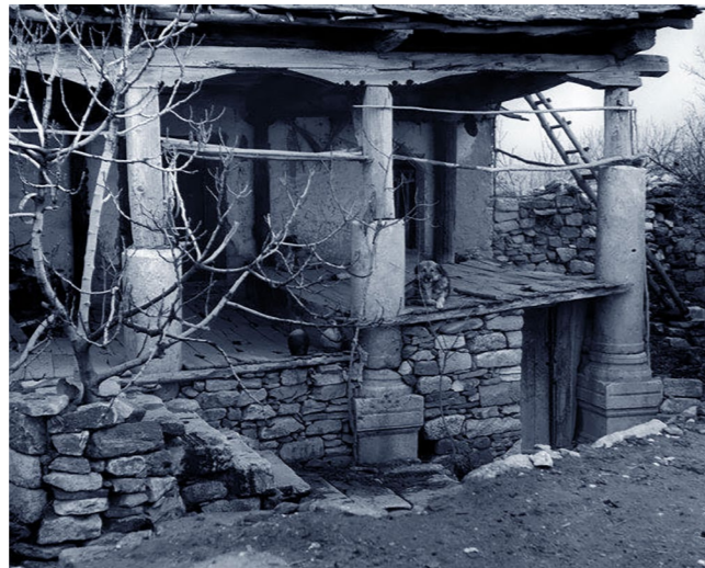
Figure 4. An example of spolia. Reuse of ancient building elements centuries later in a village house. Aphrodisias, Aydın, Turkey (Ertuğrul, E. (2021). Ara Güler'in Gözünden Tüm Ayrıntılarıyla Aphrodisias 1958. Retrieved from https://arkeofili.com/ara-gulerin-gozunden-tum-ayrintilariyla-aphrodisias-1958/ ). Photographer: Ara Güler
