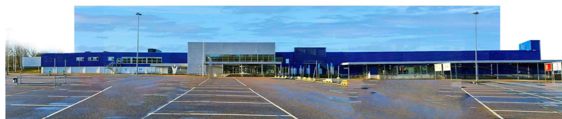
Figure 10. Current view of the east (entrance) facade, 2023.
