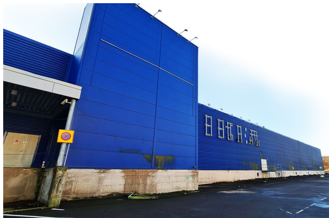
Figure 11. Current view of the north facade, 2023.
