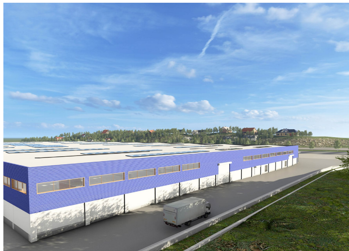
Figure 44. View of the new road and the south facade.
