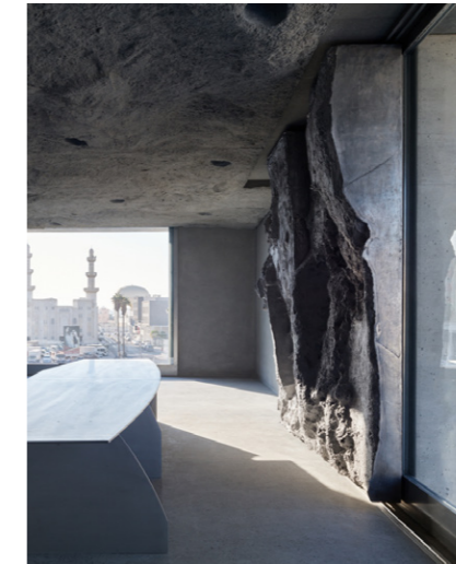
Fig 7. Sand casted concrete element. 35 Green Corner Building, Studio Anne Holtrop, 2020
