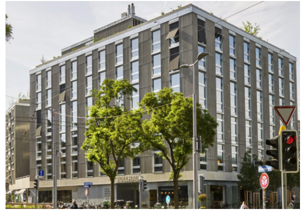
Figure 18. Zollhaus building (Martina Meier, n.d.)
