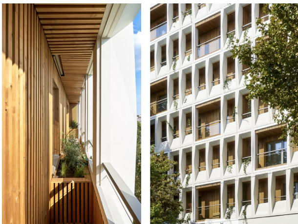
Figure 25 & 26. Transformed facade (Michel Denancé, n.d.)
