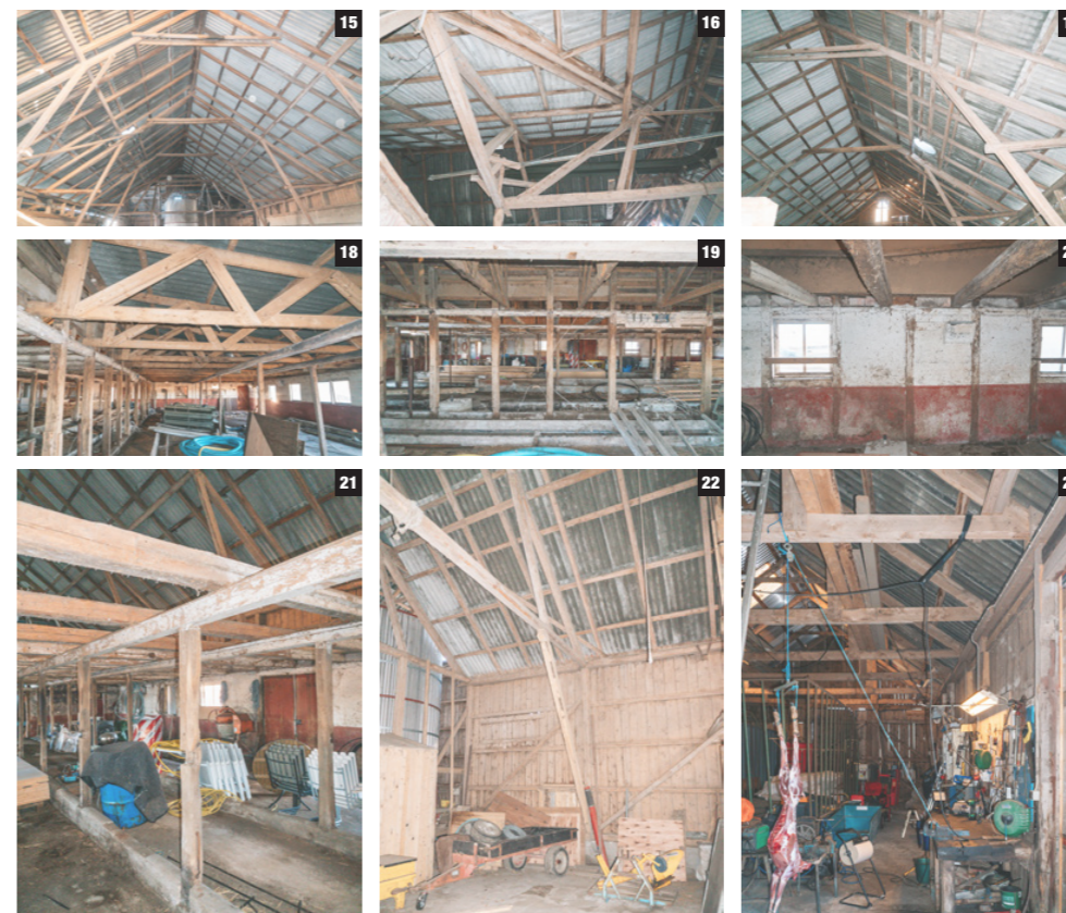
14 3d model, timber structure 15 Roof construction, wood & corrugated metal, cow house, 1930 16 Connection of cow house & silo storage, 1930 17 Roof construction, wood & corrugated metal, cow house, 1930 18 Roof construction, wood & corrugated metal, pig house, 1970 19 Interior wall structure, wood, pig house & cow house, 1970 20 Wall meeting hay loft structure, wood & brick, cow house, 1930 21 Hay loft structure, wood & concrete, cow house, 1930 22 Roof structure meeting wall & floor, wood & concrete, 1930 23 Roof / wall structure, wood & concrete, brew house 1970
