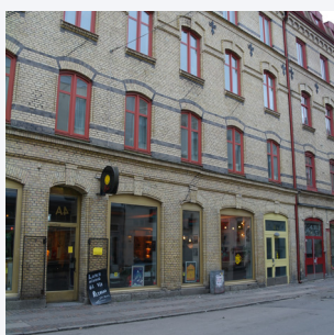
NO PROTECTED SPACE ALONG THE FACADE, BUT A CONNECTION TO THE INSIDE
