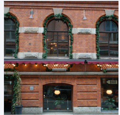
Visual connection between the sidewalk and inside with low basement windows.
