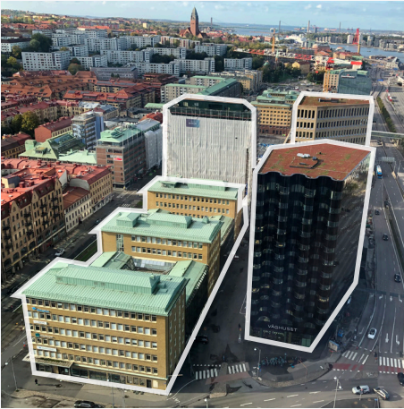
MASTHUGGSKAJEN HAS LARGE PLOT GRAIN WHICH LEADS TO LESS VARIETY IN FUNCTION AND VISUAL EXPRESSION ALONG THE STREET
