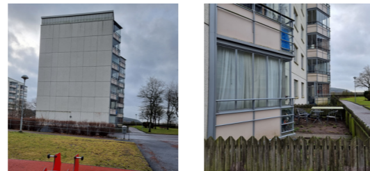
Fig. 58. Windowless façade and closed blinds.
