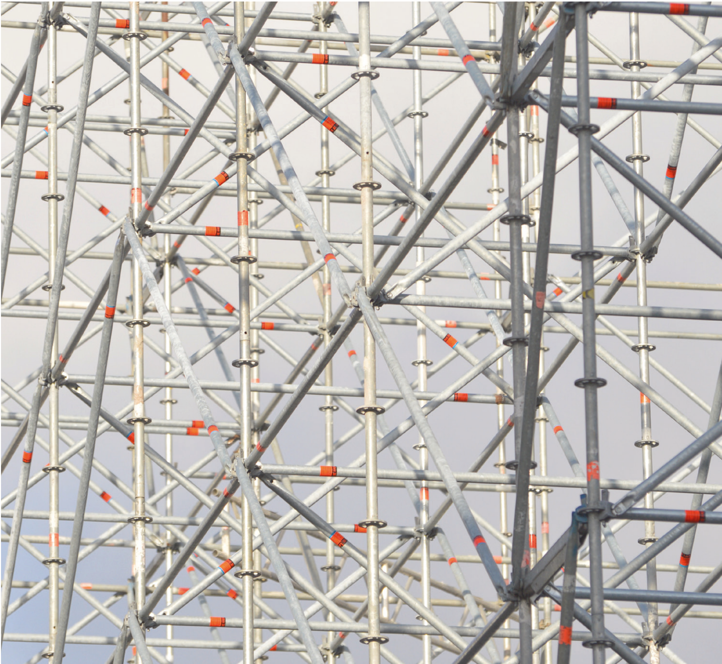
Fig. 02. Construction scaffolding in Göteborg
