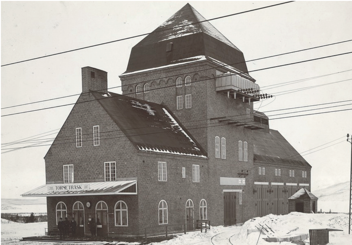
Figure 5: Torneträsk station house and transformer, 1914
