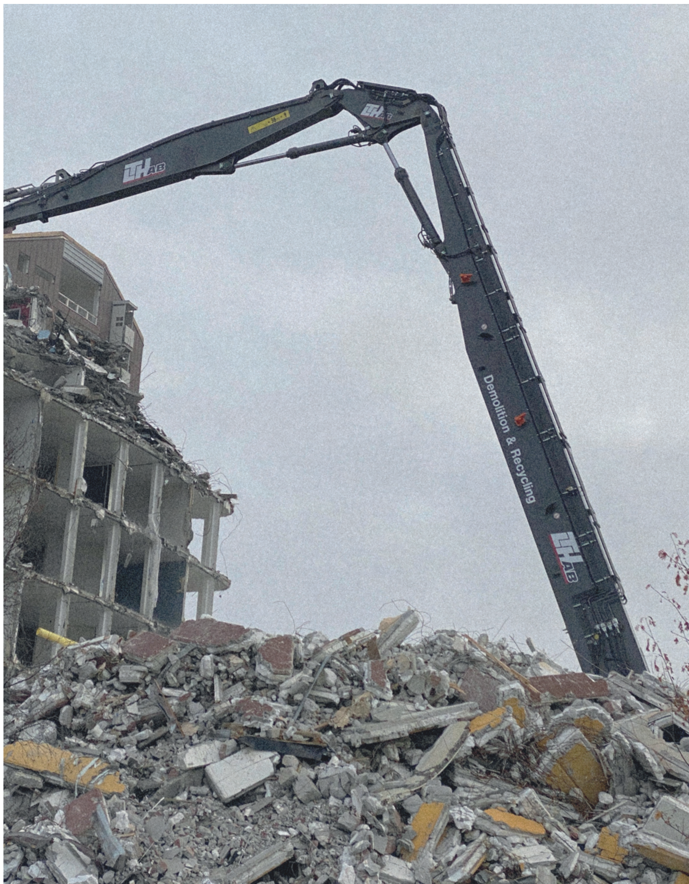
Ordrivaren by Ralph Erskine being demolished in Kiruna
