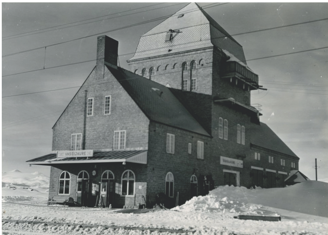
Figure 6: Vassijaure station house and transformer, 1915
