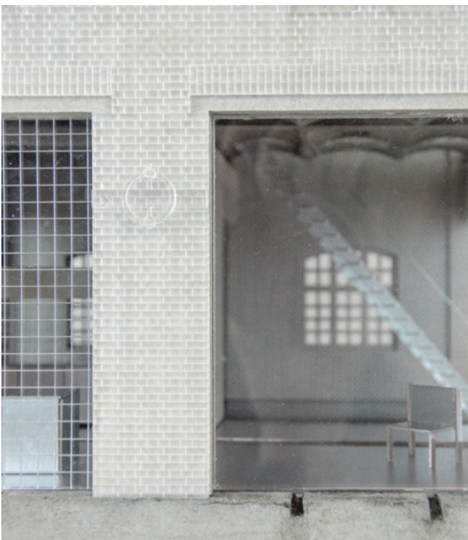
Replaced doors creating a permeable facade
