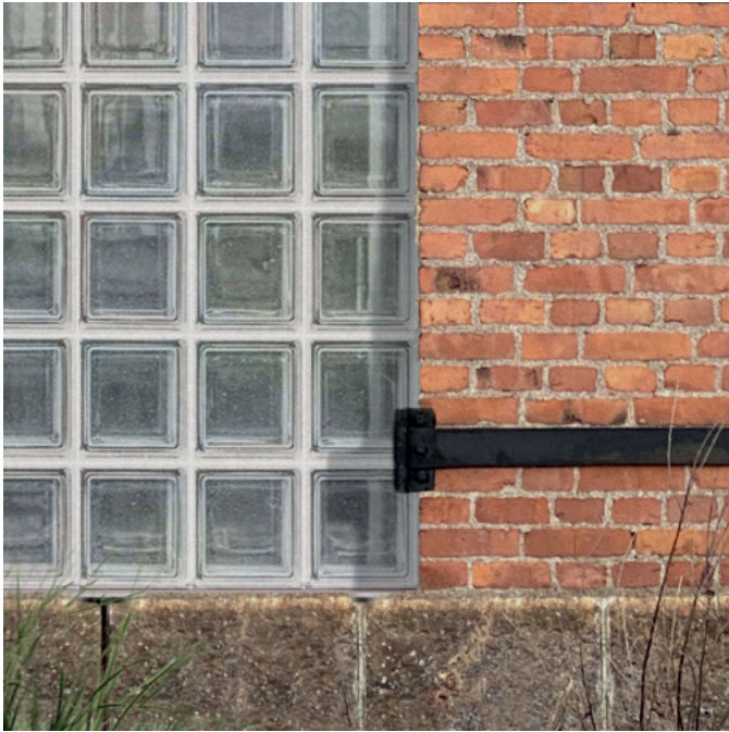
New glass concrete meets original brickwork
