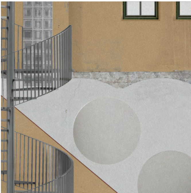
Trace of subtracted joist in relation to an added stair
