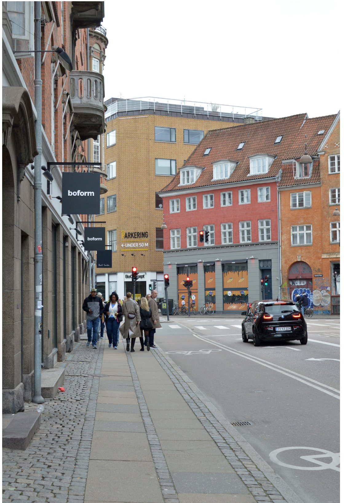
The textile quality of the facade appears in the neighborhood scale.
