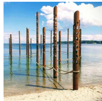
Personal communication (January 23, 2024). Photo showing the facility up close and the corten steel material on the pillars. [Photograph].
