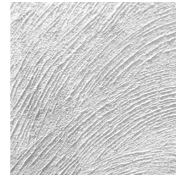
SEALAB (n.d.). Three examples showing different wall structures used in the building. The texture help the user to navigate. [Photograph]. https://www.sea-lab.org/School-for-blind-and-visually-impaired-children
