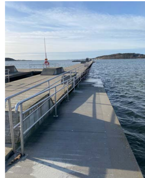
Figure 43: Photo of ramp.
