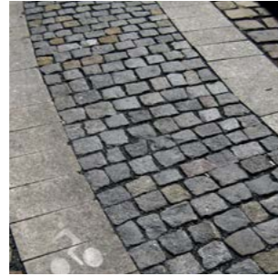
Figure 14: Main path in lighter pavement tiles, for better visibility.
