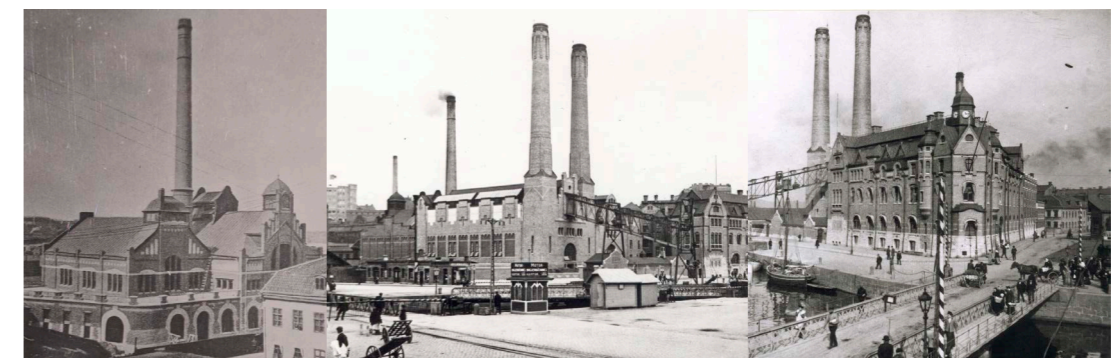
The Previous Power Station Design by Hans Hedlund from Early 20th Century Left: Tram Power Station, 1902; Mid: The Power Plant with The New Coal Elevator, 1908; Right: The Newly Constructed Office Building, 1903 (Energihistoriska samlingarna)
