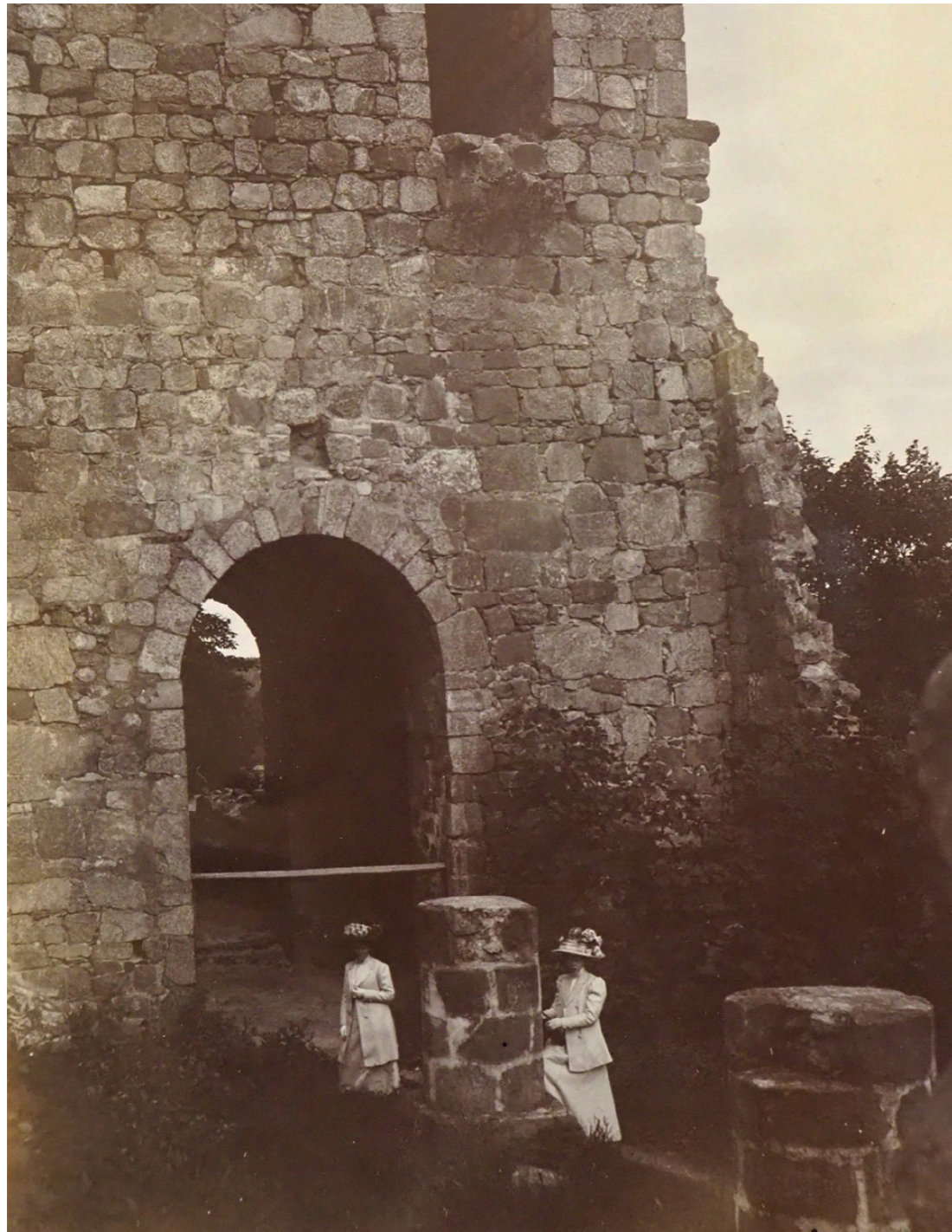
The ruin is explored by two women after the 1890s restoration. The masonry is secured and the central pillars bricked up to an even level. Vegetation still occurs inside the nave. E Eckhoff, 1890s. Source: Bjerking AB. (2020, June 23). St Per - restaurering. p.4.
