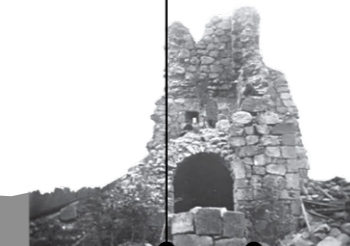
St. Per before Ekhoff's restoration in 1895
