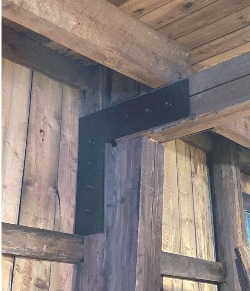
Recent structural addition on the ground floor
