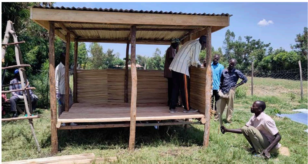
Figure 33: Man trimming the papyrus reed mat used as insulation
