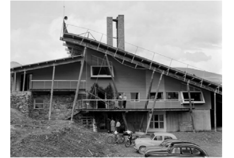
1954- building of Borgafjäll Hotell by Ralph Erskine.
