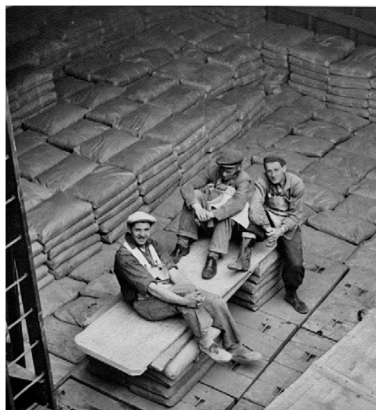
Loading of cementsacks on a ship, 1949 Unknown photographer accessed through Othem-Boge Hembygdsvörening
