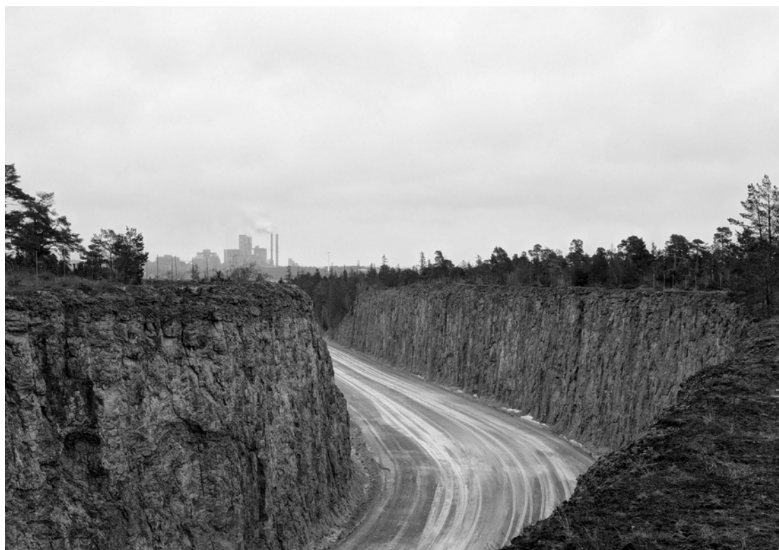
Cementplant and Truckroad connecting Västra brottet & File Hajdar
