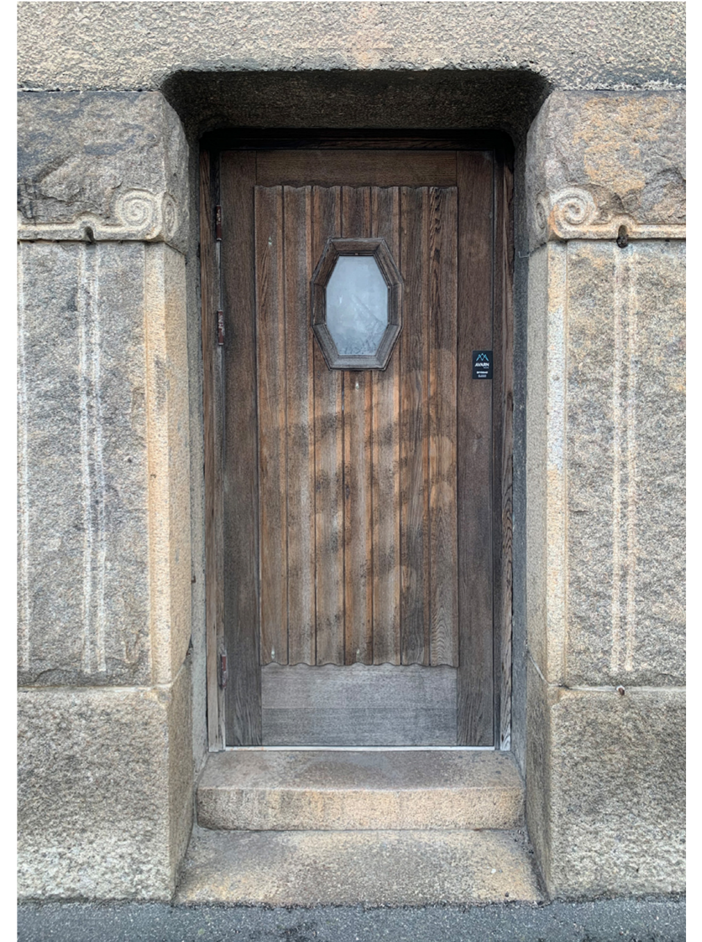
blocked former entrance of skeppsbron 4
